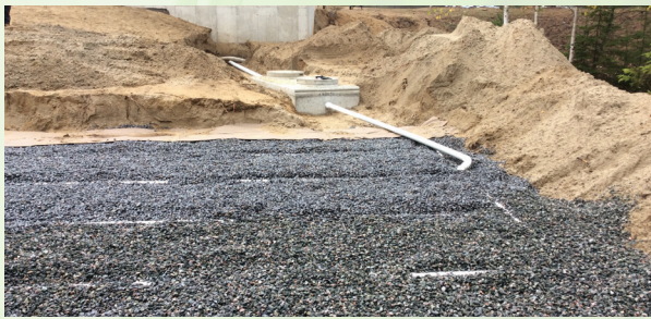
Septic tank (cement reservoir) followed by a septic field (a type of soil absorption system).
