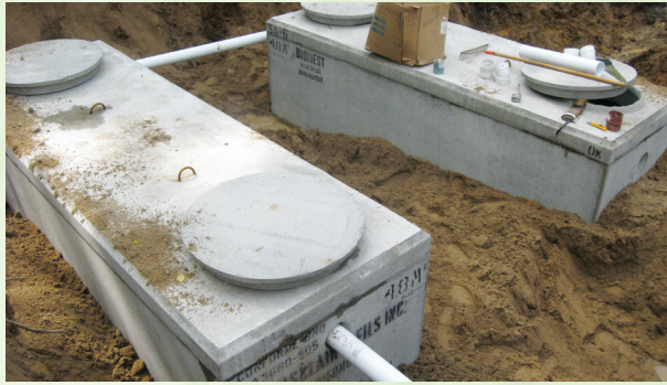
A septic tank followed by a Bionest. The Bionest reservoir is very similar to the septic tank.
