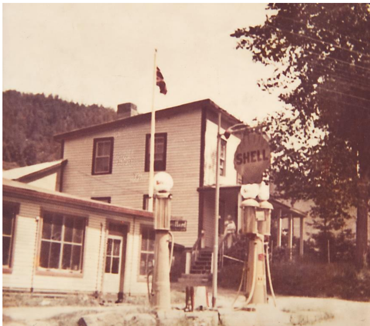
Rosario Matte's first garage, photographed in 1947. Razed by fire in 1960, the building was rebuilt, and then renovated in 1998. Source: Matte family collection, photographer unknown.
